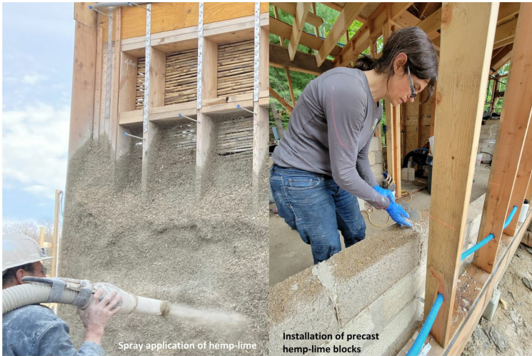
Spray application of hemp-lime
