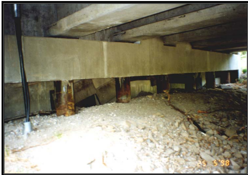
Exposed Bridge Abutments at the Little Chena River
